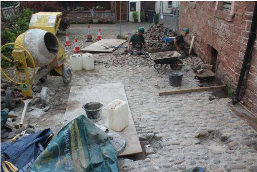
Relaying the yard cobbles on the east side of the barn
