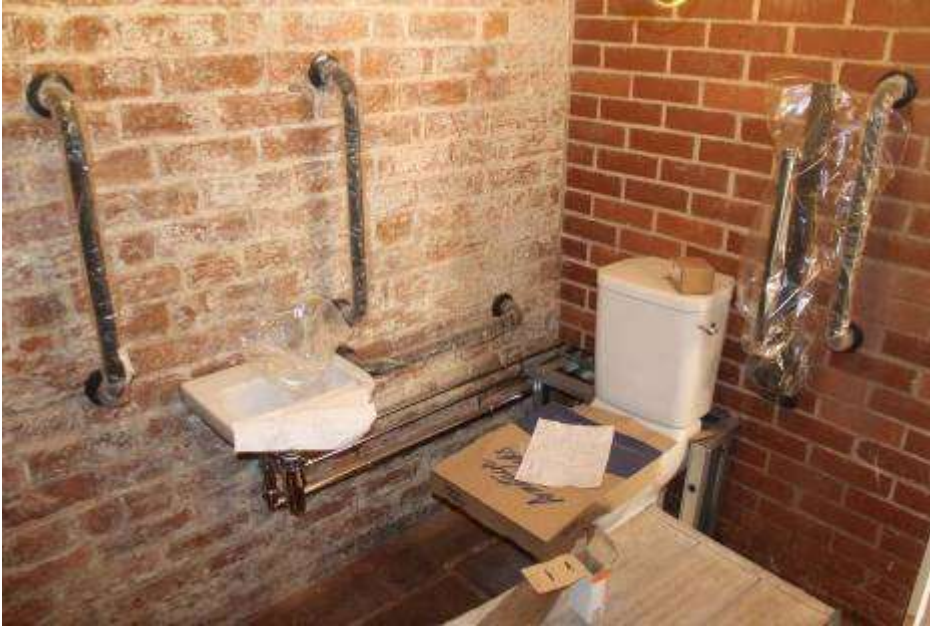
Fitting sink and toilet in the old ground floor store
