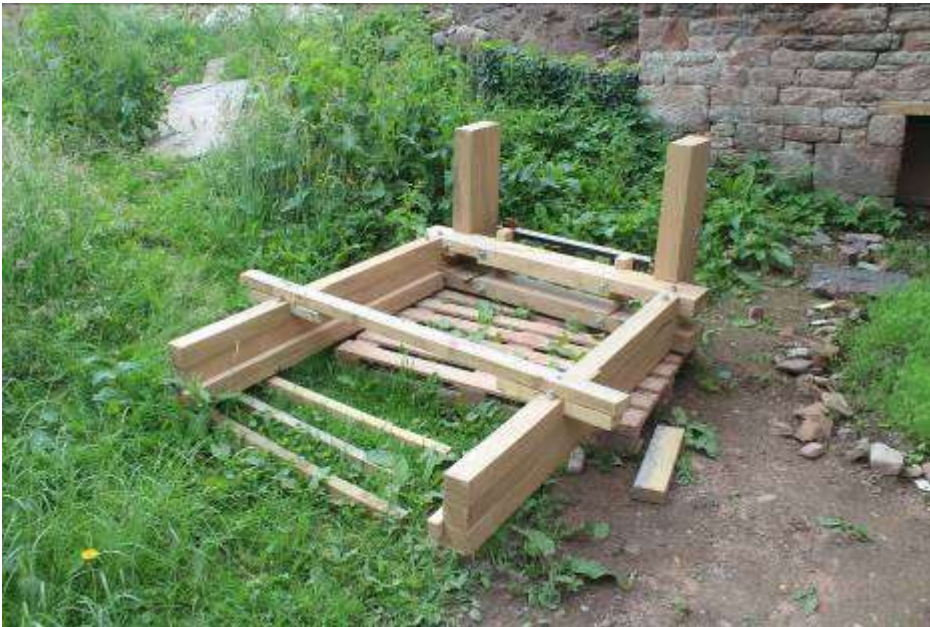
The framework of the new escape sluice arrives on site
