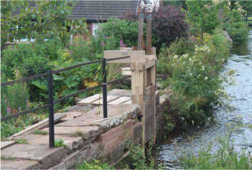
Looking upstream towards the new escape sluice
