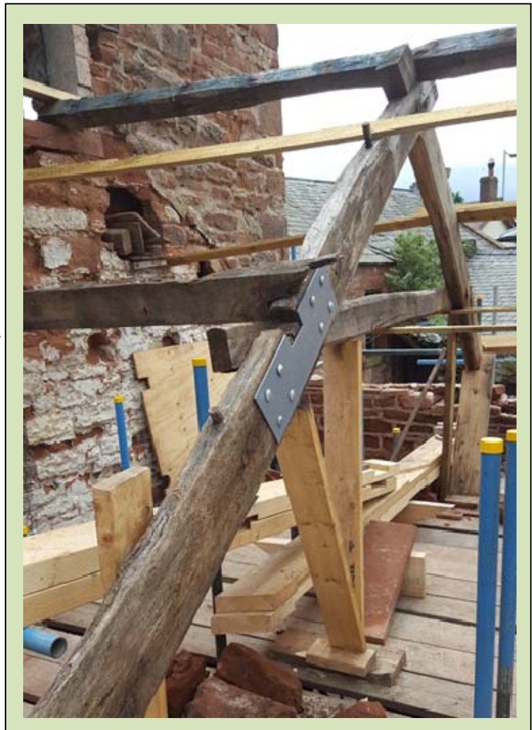
A bespoke metal plate repair to an existing roof truss.
