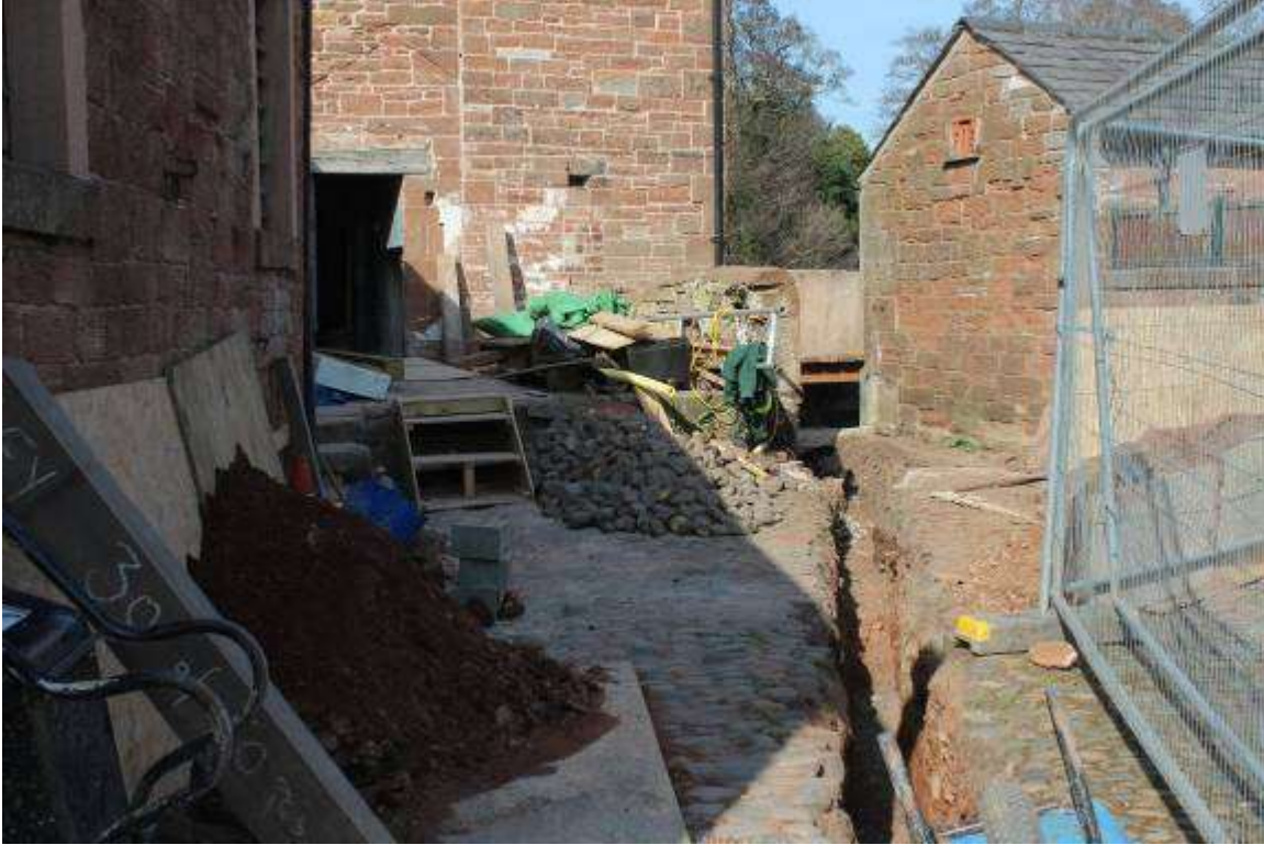
Drain crossing the yard to the east of the barn
