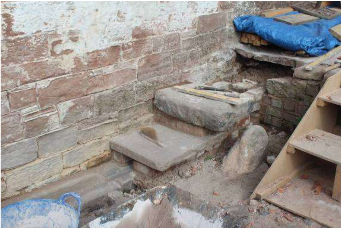
Reinstating the steps up to the loading dock
