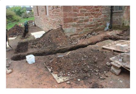
Since March, the main external works have been to identify suitable locations for the drainage trenches and incoming power and water supplies for mill – this has meant several test trenches being opened up to ensure sufficient depth to allow the services to be safely located. A few places were tested – uncovering glimpses of earlier cobbled yards and foundations of structures but eventually suitable locations were found.
