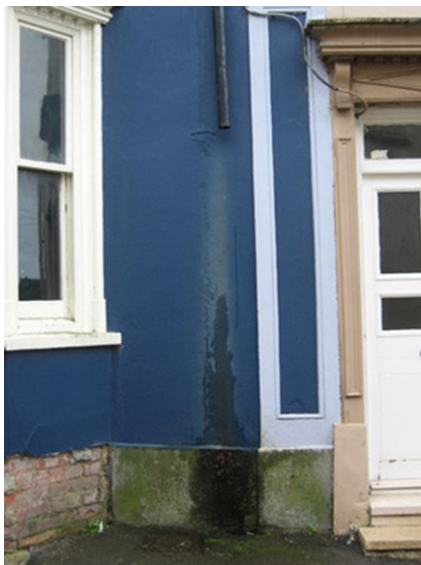
Missing downpipe
