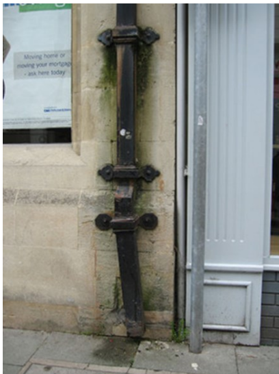
Broken downpipe
