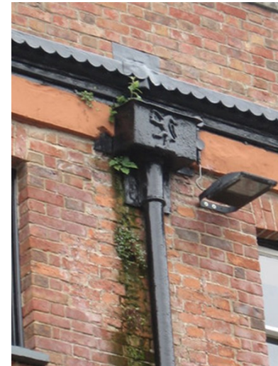
Blocked downpipe
