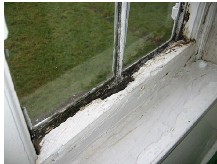
Rotting woodwork
