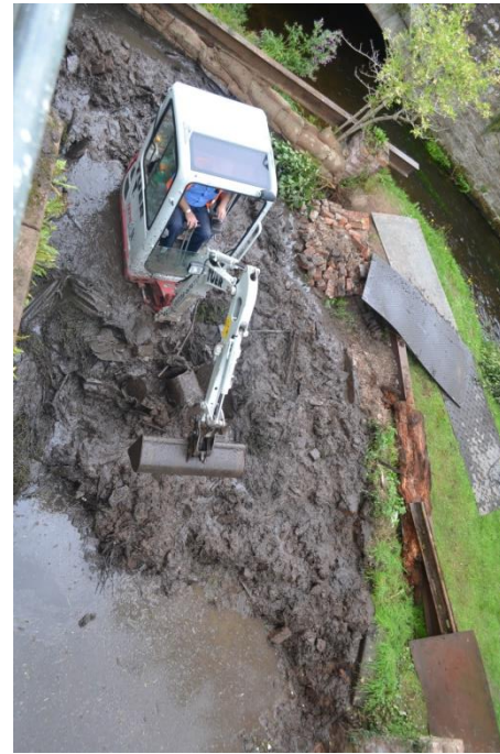
Figure 12 Clearing nearly 30 years of silt and debris from the tailrace
