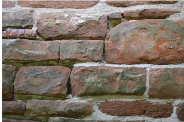
Figure 14 and 16 checking alignment of new stone inserted above a window opening and close up of new lime mortar pointing in north wall
