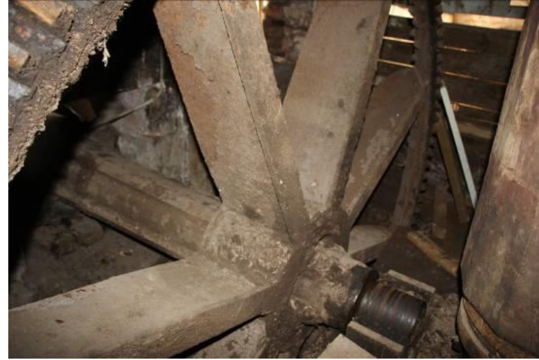
Figure 5 Fine silt removed from the headrace and the remaining buckets removed from the wheel [Photo Harry Beamish, Archaeologist]
