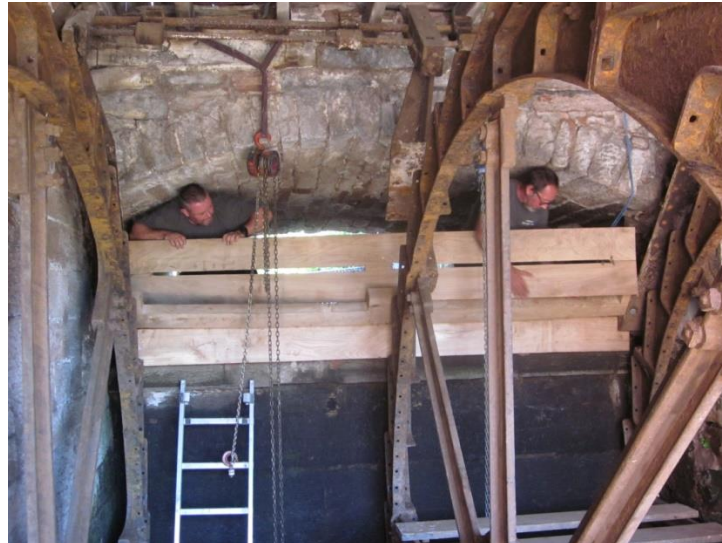
Figure 4 Fitting the Control gate in position to direct the water into the wheel buckets
