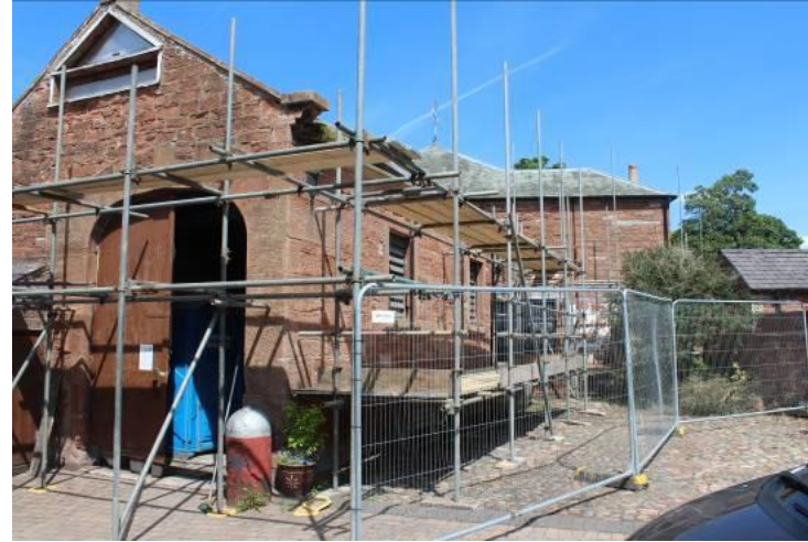
Figure 10 Scaffold erected around the barn to allow access to inspect the stonework
