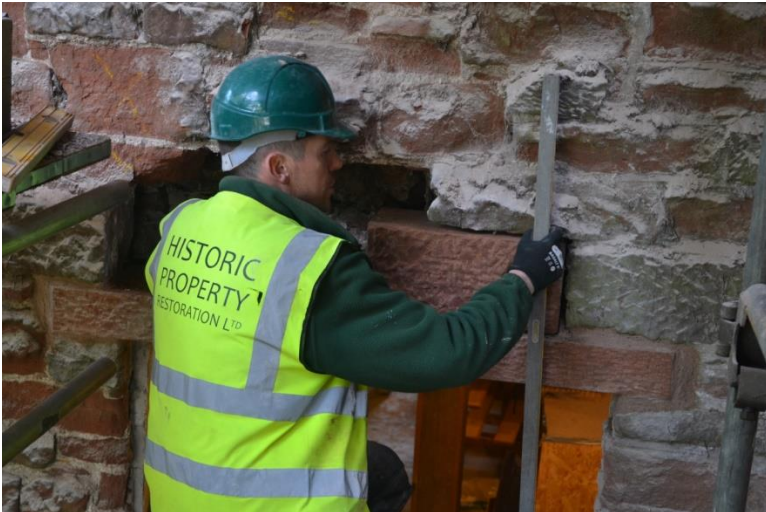
Figure 14 and 16 checking alignment of new stone inserted above a window opening and close up of new lime mortar pointing in north wall
