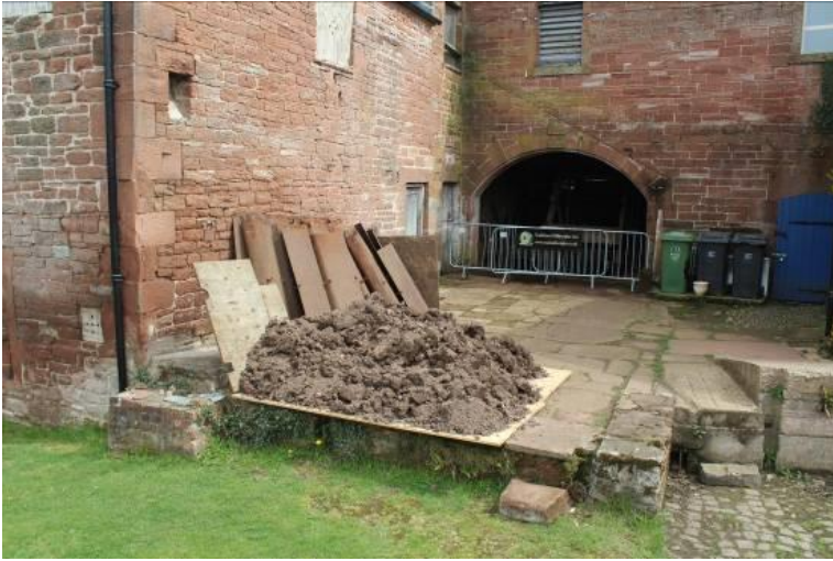
Figure 5 Fine silt removed from the headrace and the remaining buckets removed from the wheel [Photo Harry Beamish, Archaeologist]
