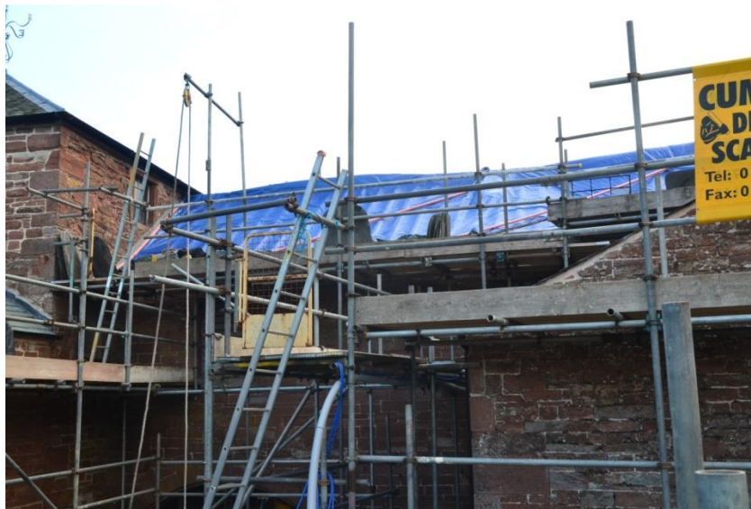
Figure 16 Slates removed from barn roof and tarpaulin in place
