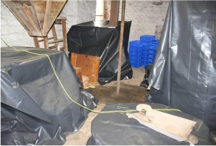
Figure 9 Protecting millstones in advance of building repairs
