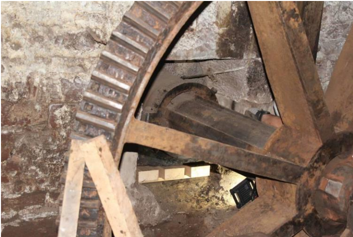
Figure 7 new packing blocks being inserted below the centre bearing of the waterwheel
