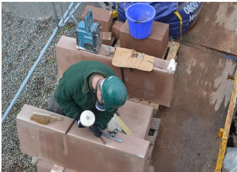
Figure 15 hand carving new coping stone for top of tailrace wall
