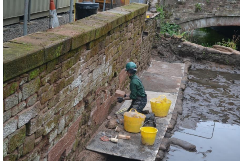
Figure 13 Tail race with sandbags in place, commencing cleaning of stonework to identify repair/repointing required and Fig 14, Mason fitting hand chiselled stones into place
