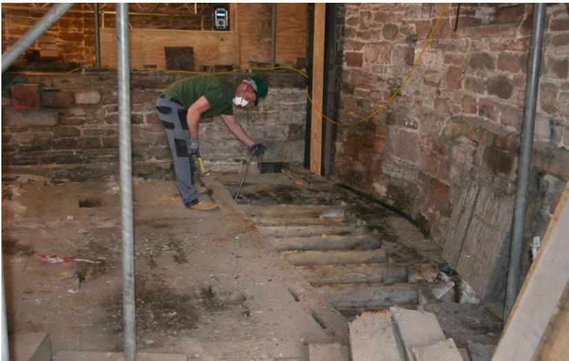
Figure 11 Checking the joist ends for damage and structural integrity
