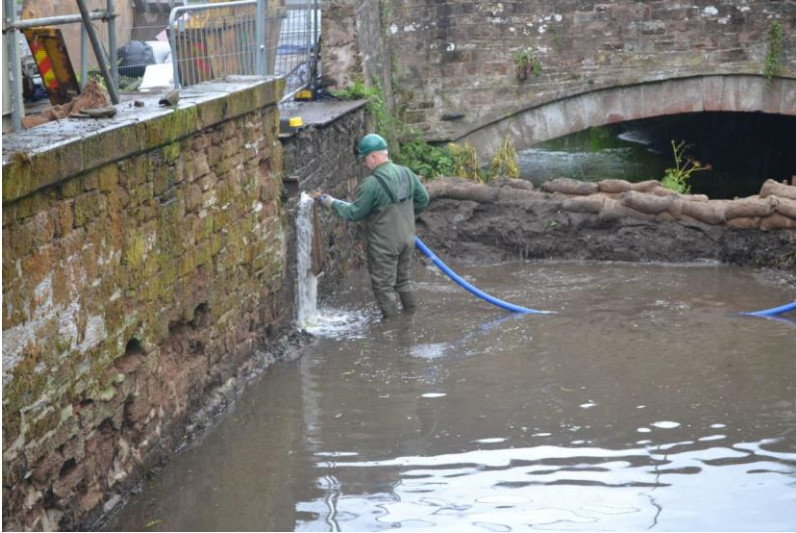
Figure 13 Tail race with sandbags in place, commencing cleaning of stonework to identify repair/repointing required and Fig 14, Mason fitting hand chiselled stones into place
