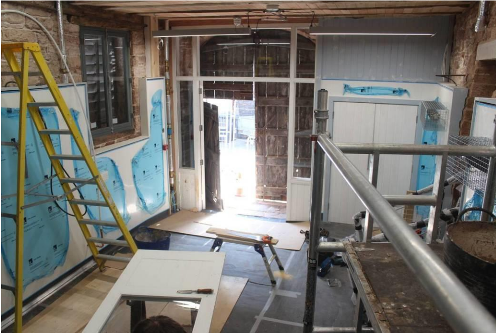
Looking south inside the barn
