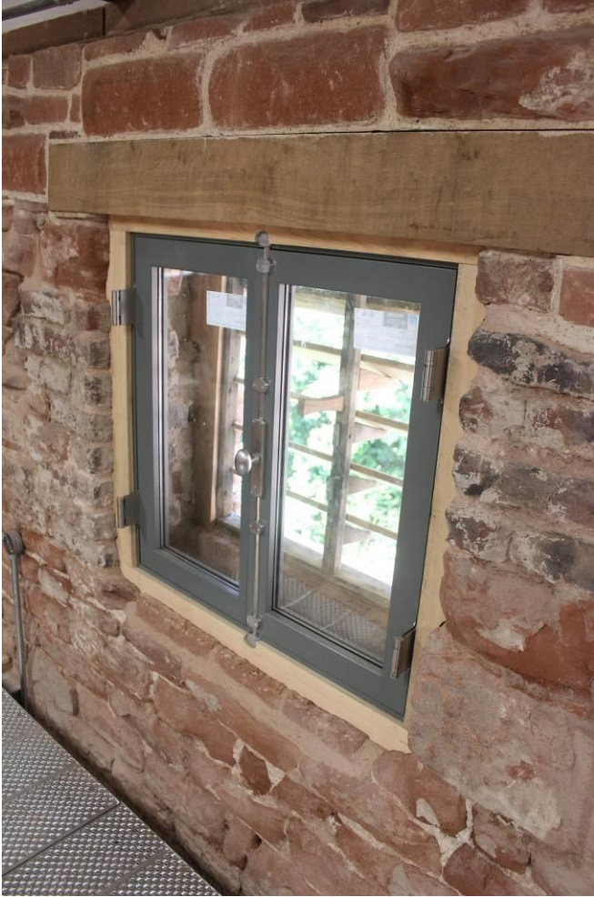
Secondary glazing inside the refurbished shutters in the kiln building
