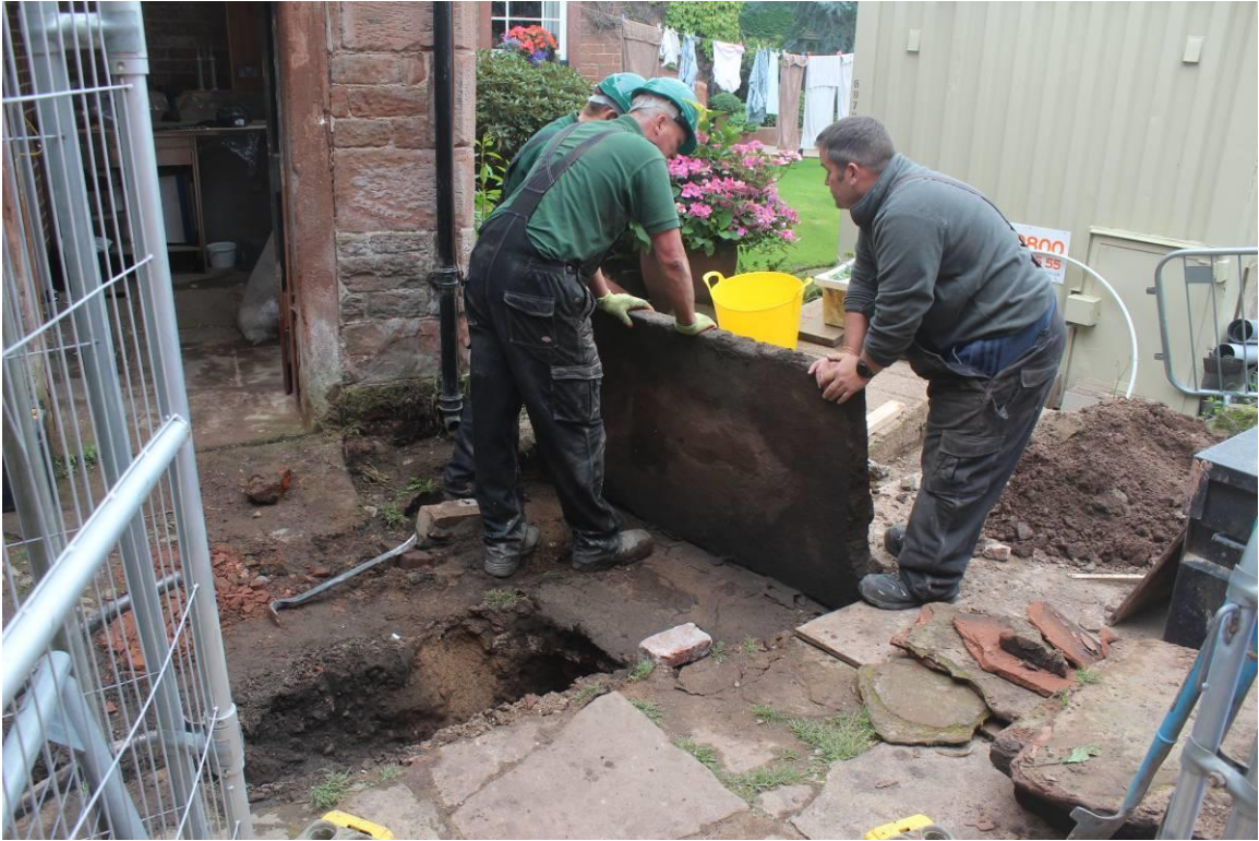
Lifting a large sandstone slab on the line of the drain
