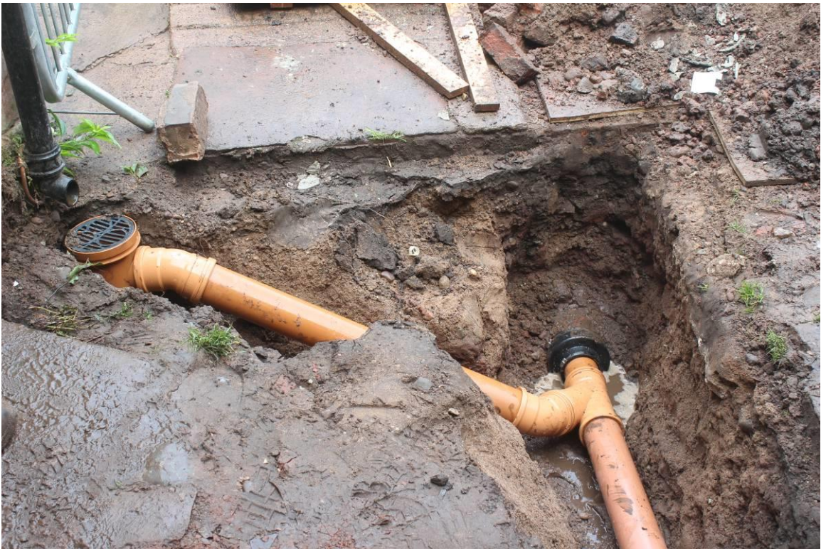
New drainage in place
