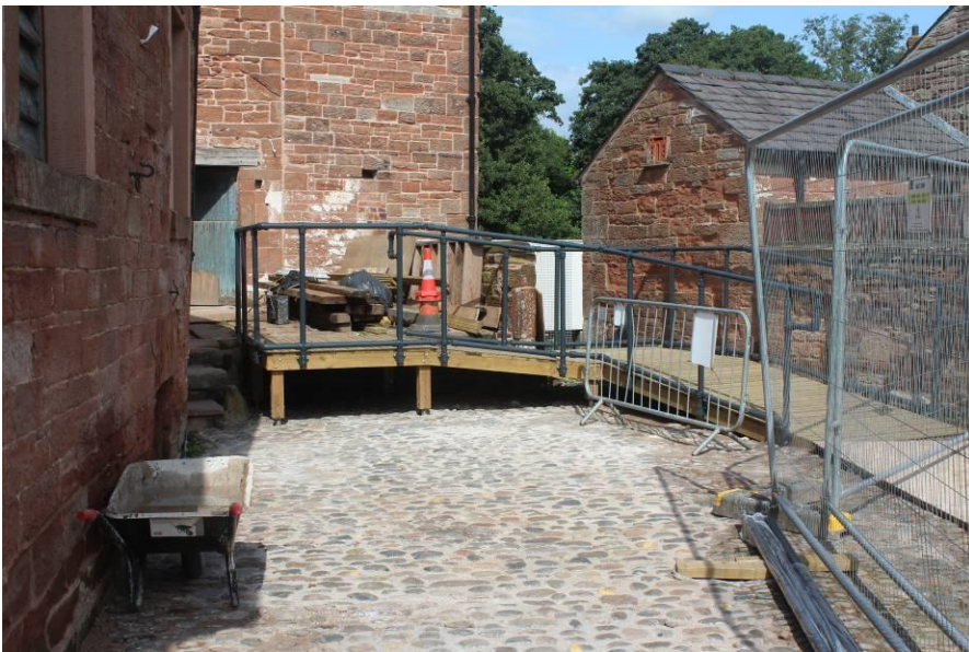
The new access ramp completed in the east yard
