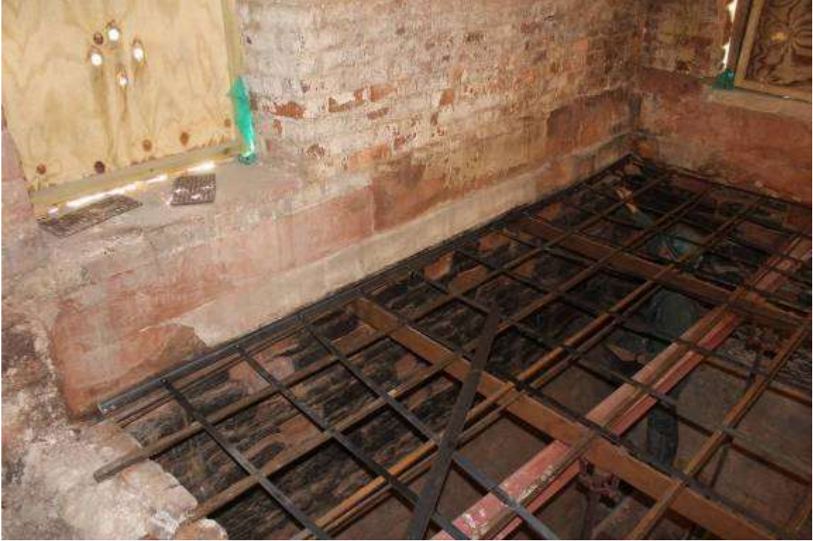
Pointing in the reinstated wrought iron bars. New ribbon partly re-instated
