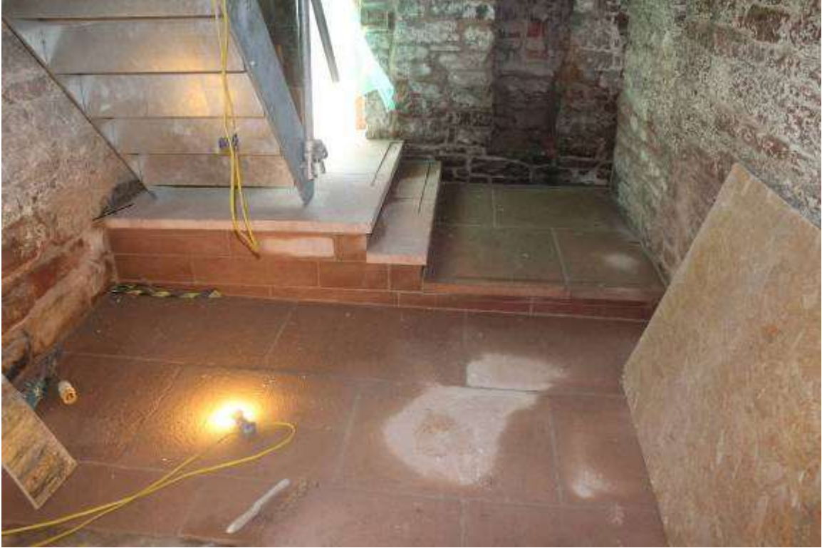
New landing, steps and floor to the east of the kiln
