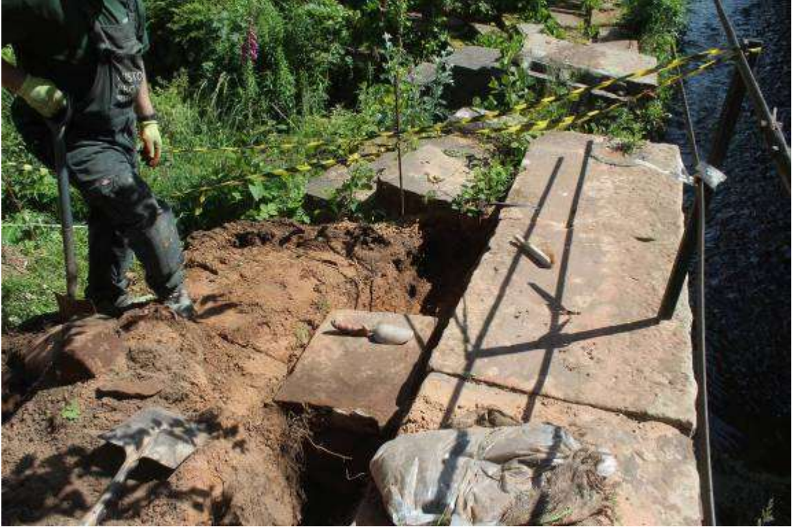
Cable trench approaching the escape sluice position
