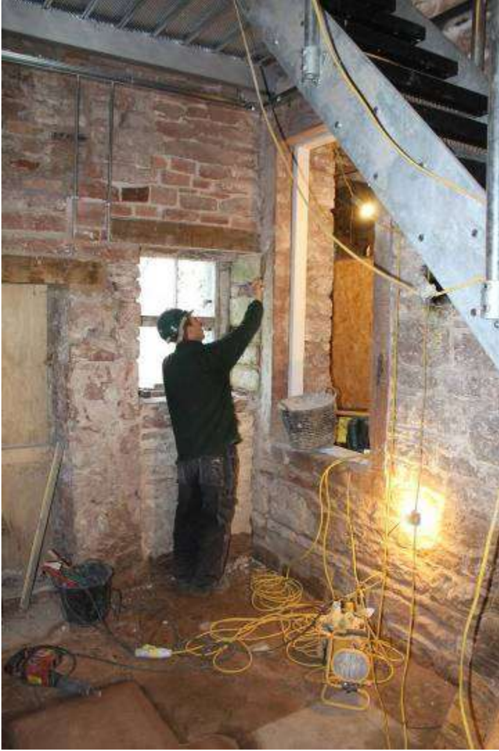
Pointing around window opening in the kiln
