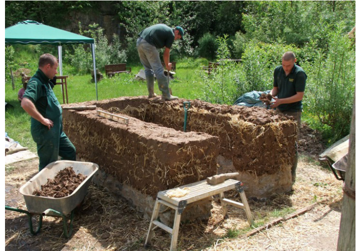
Applying the layers of dabbin mix, building onto the plinth
