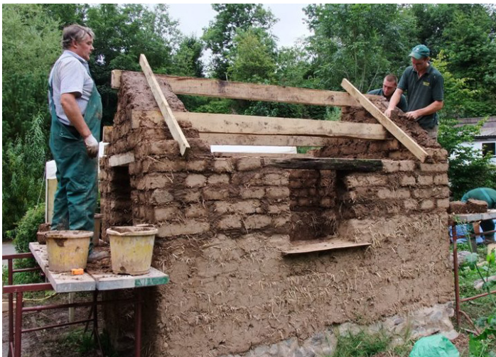
Adobe blocks above the layered dabbin mix
