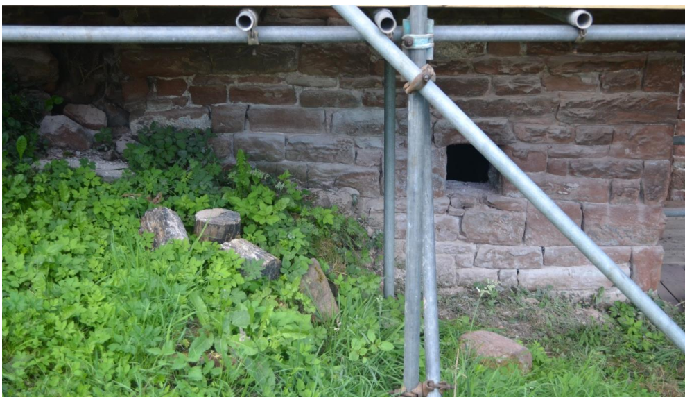
Figure 2 Section of wall with old mortar removed ready for repointing
