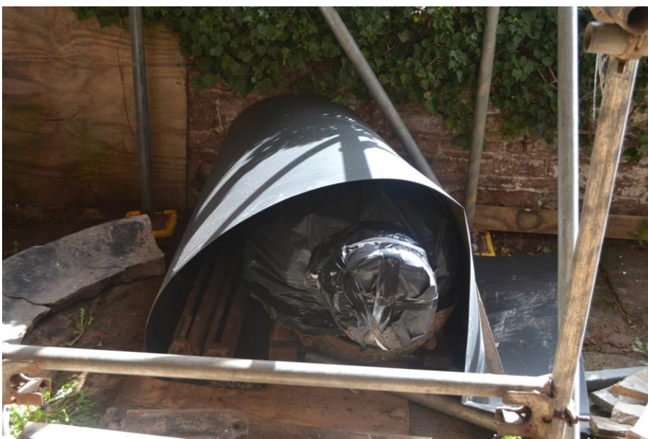
Figure 6 Large electric motor moved from tower and protected
