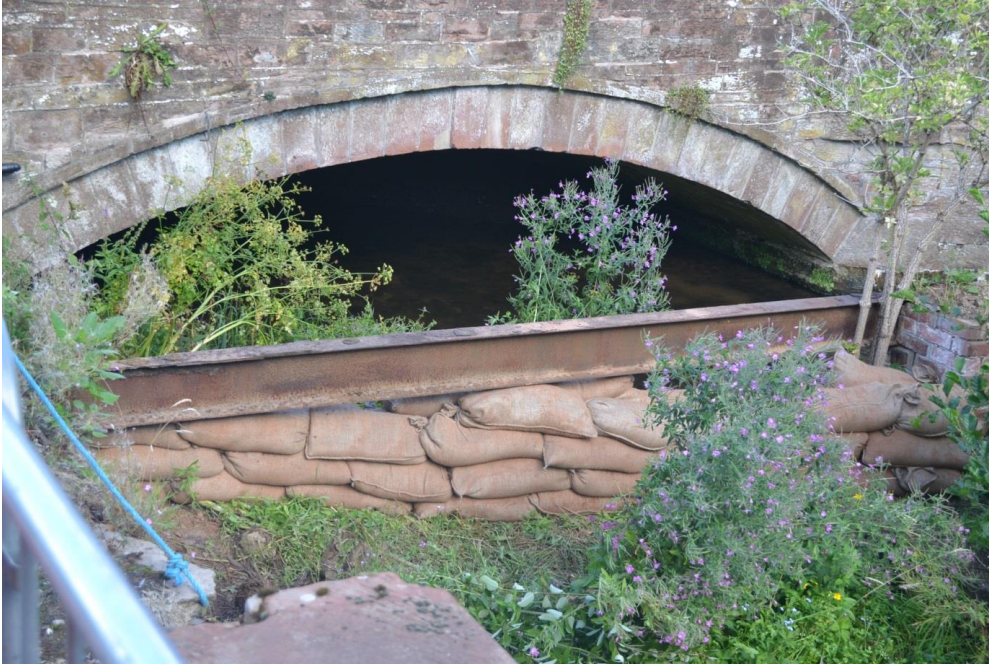
Figure 1 Cofferdam in place to prevent back flow of water from the river into the tailrace
