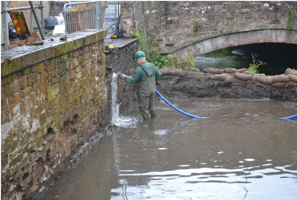
Figure 5 cleaning stonework in tailrace
