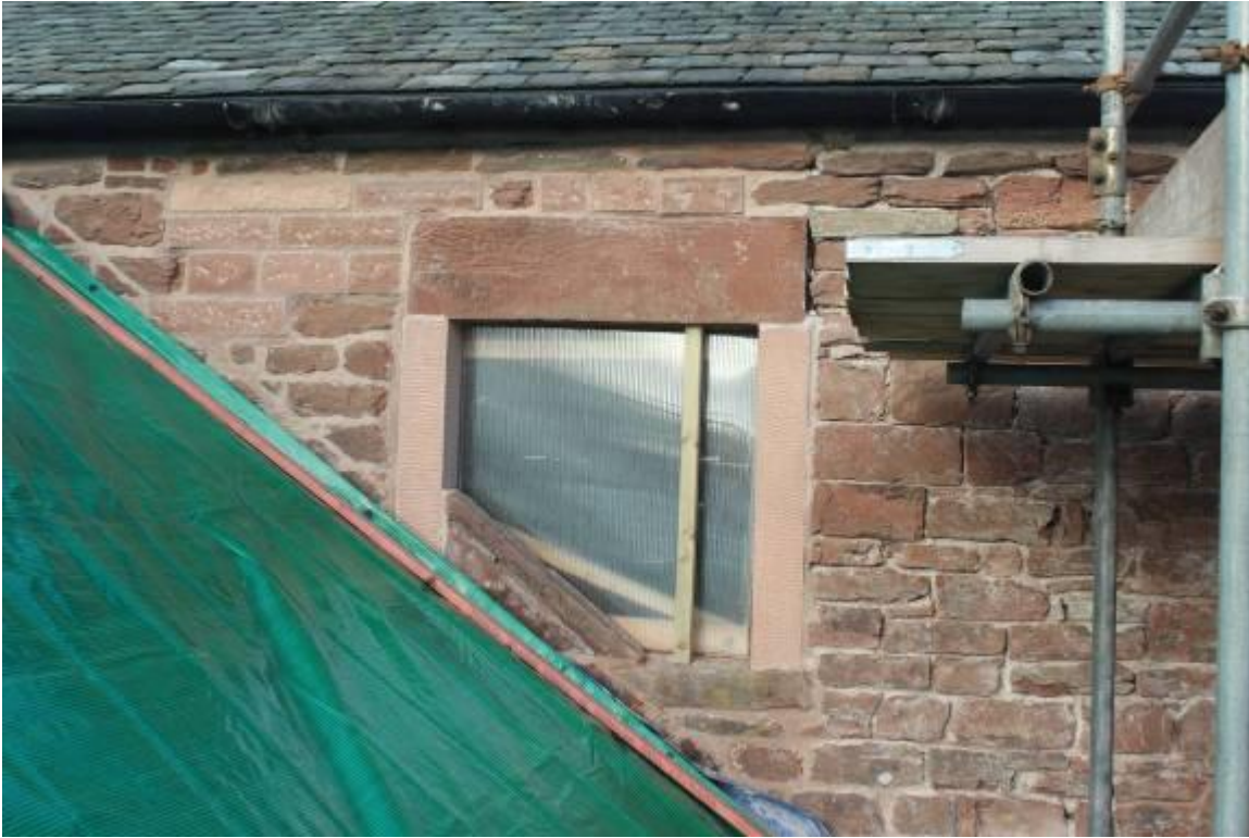
New jambs replacing failed stones at the shutter opening in the south wall of the mill at Garner Floor level. The opening was cut across when the threshing barn was added to the 1839 mill building
