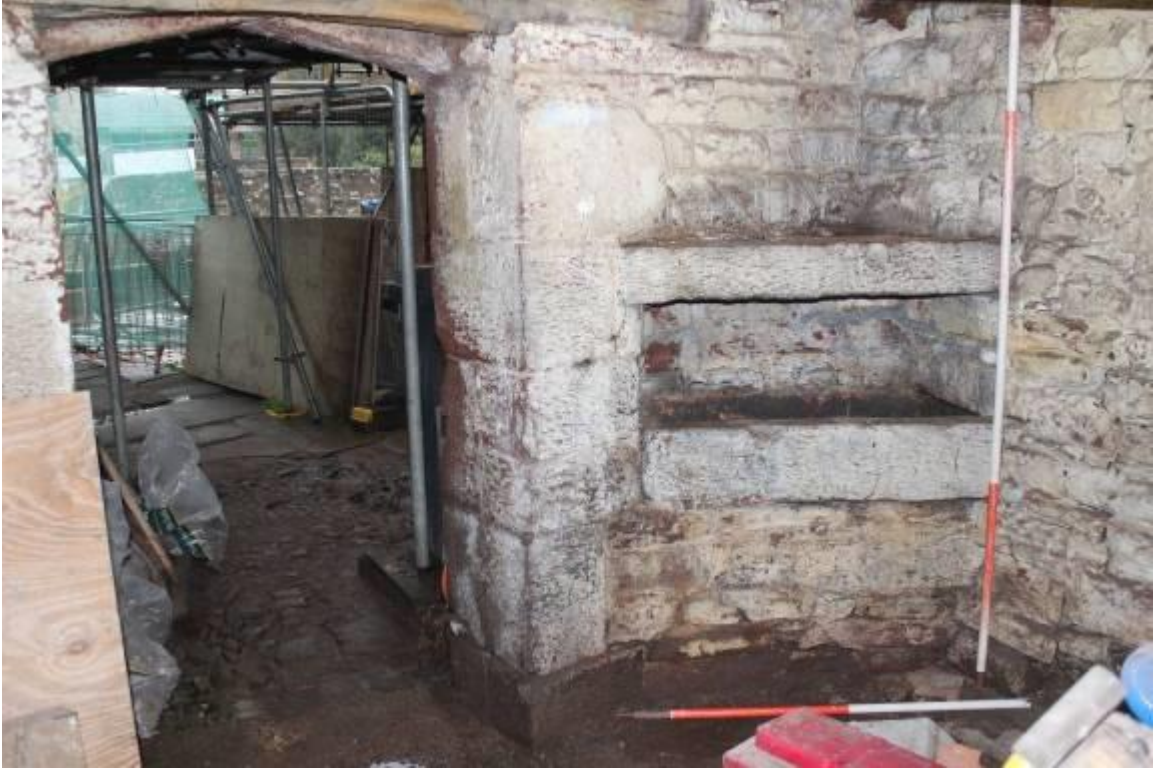
A nicely executed stone trough in the NW corner of the store with a substantial slab above – perhaps acting as a tie across the vulnerable external angle of the earlier range?
