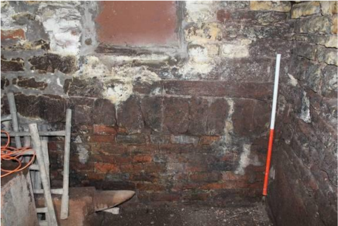
A nicely executed stone trough in the NW corner of the store with a substantial slab above – perhaps acting as a tie across the vulnerable external angle of the earlier range?
