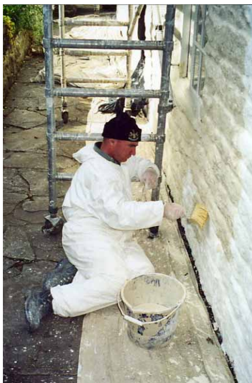
National Trust Building Team limewashing
