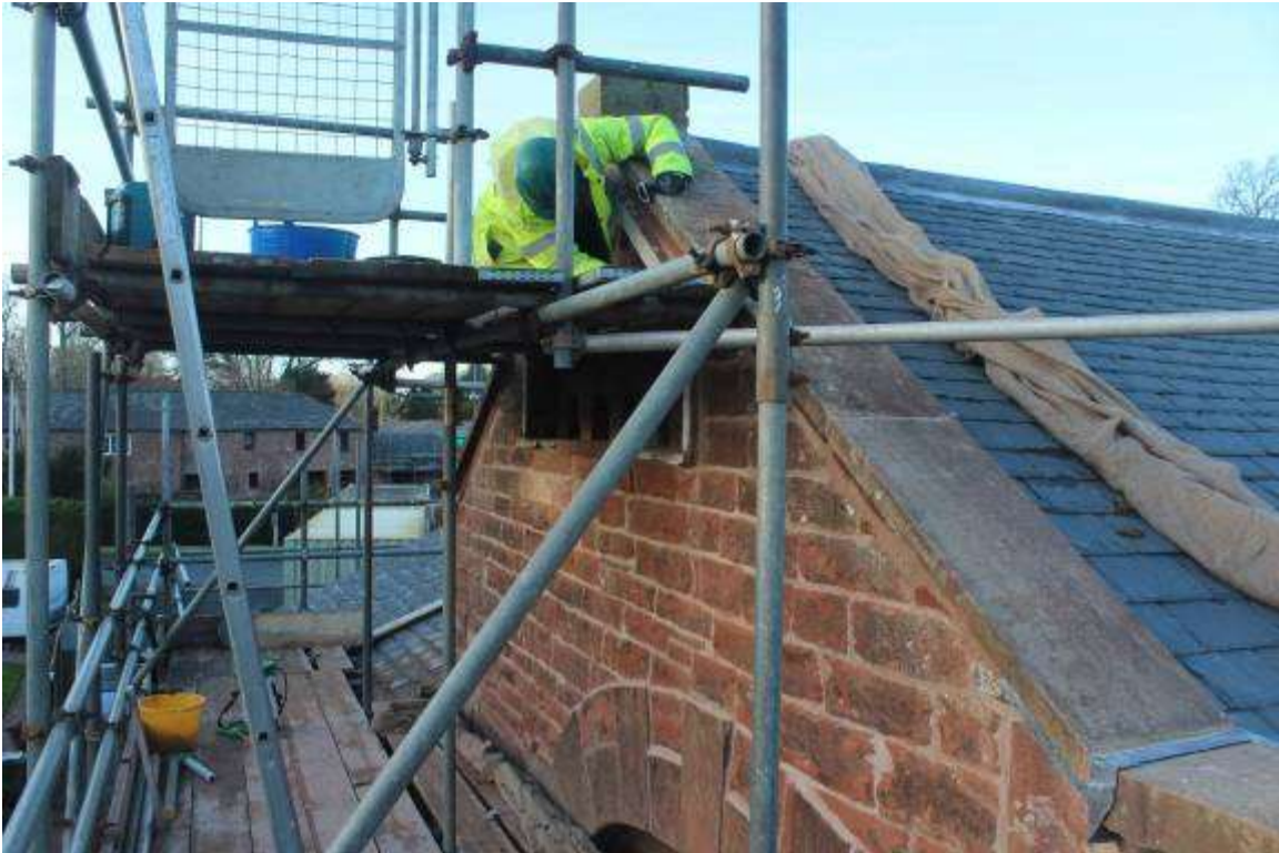
Alan putting the finishing touches to the gable of the Barn
