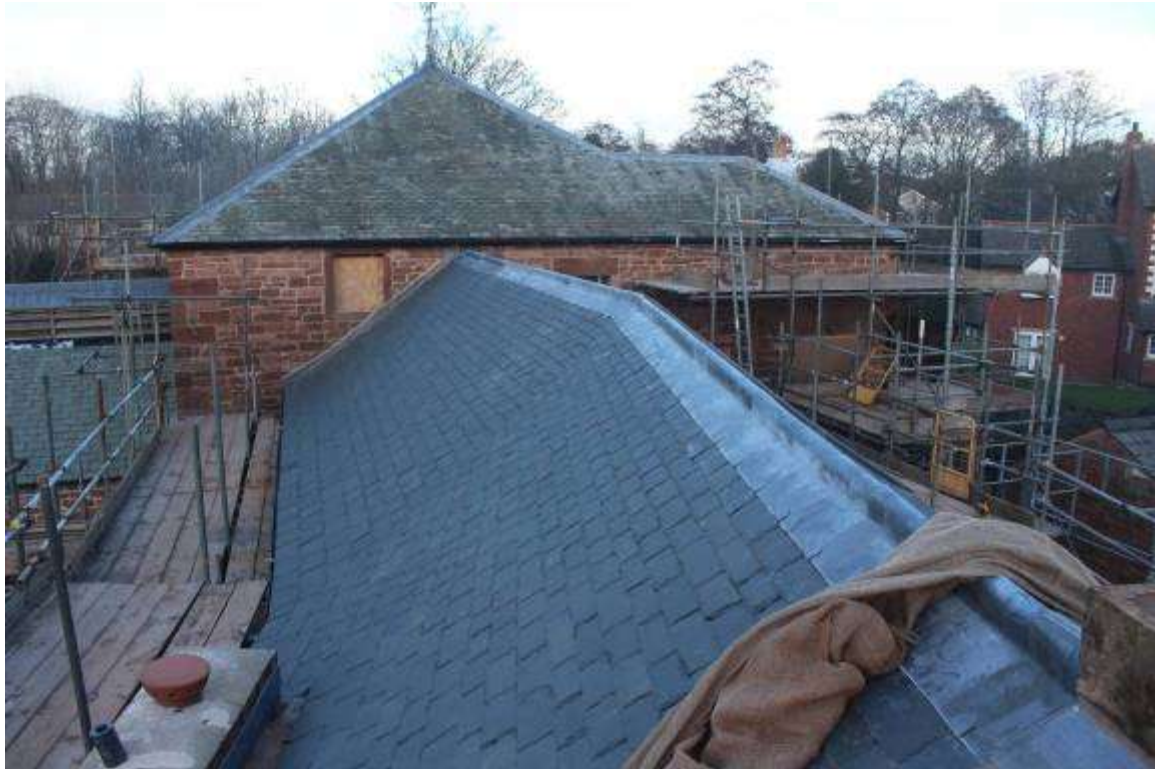
New roof on the barn completed
