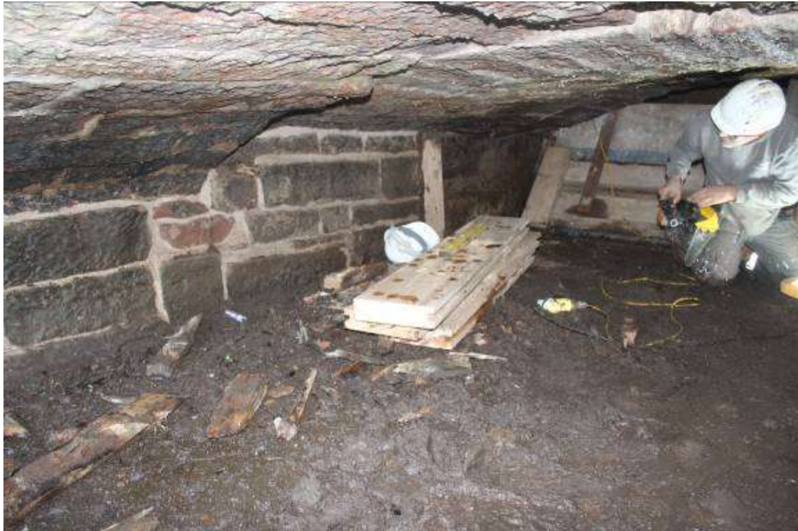
Work in progress on the south side of the culvert
