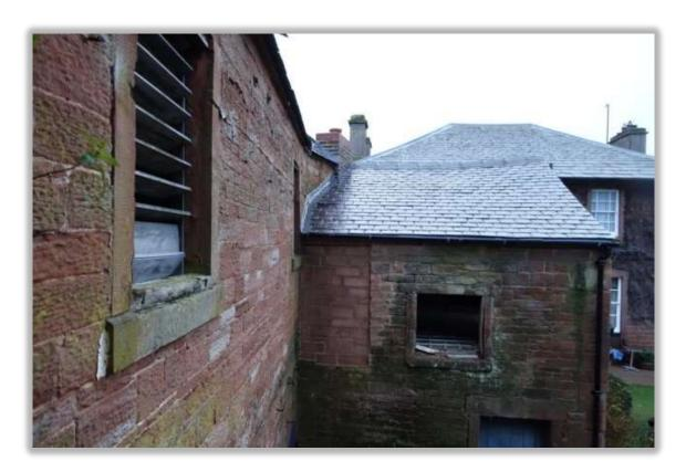
As well as the visible exterior work, some of the supporting roof timbers have been strengthened and some stone replacement and re-pointing with lime mortar has also been carried out.
