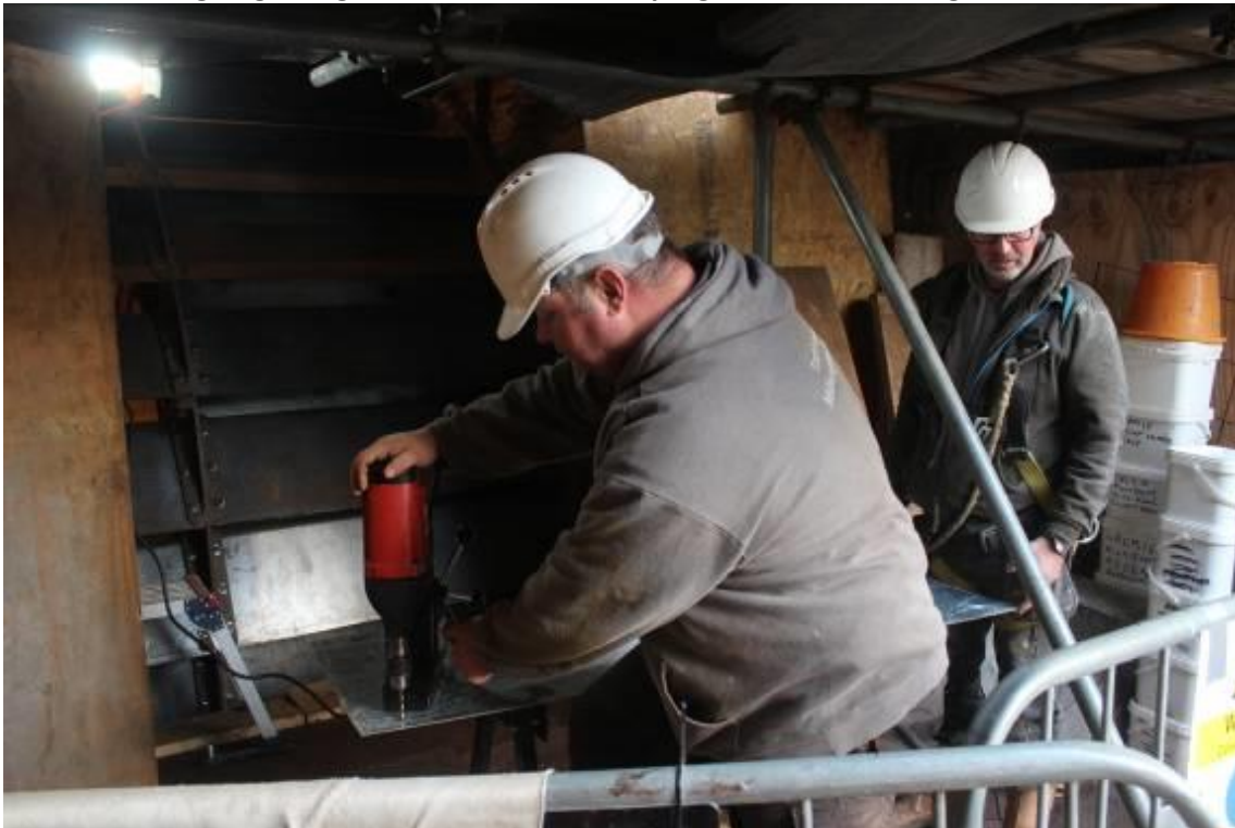
Jon drilling bolt holes in one of the new sole plates
