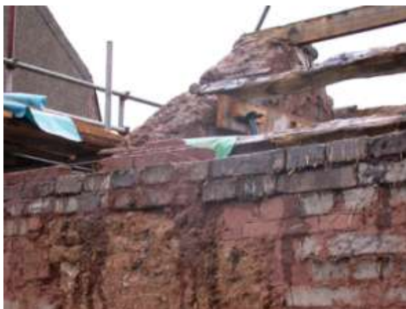
Clay blocks laid on top of the original wall to create a new wallhead
