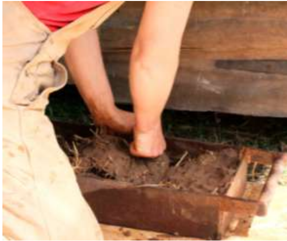
When making the clay block the mixture needs to be well compressed into the mould Drying the blocks on a flat surface
