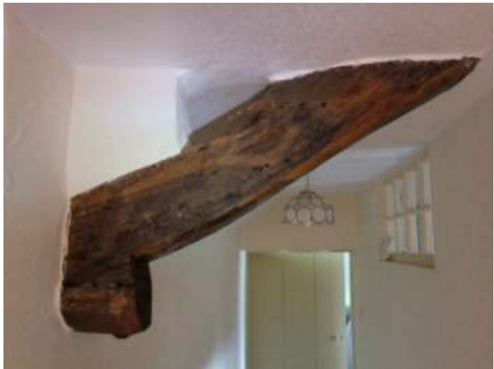
Tie-beams cut through to give headroom upstairs
