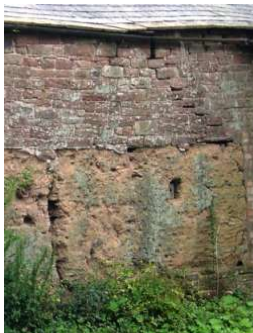
Cracking probably caused by movement in the plinth
