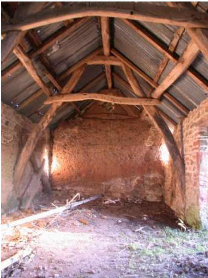
Crucks are often associated with clay dabbins. This example is on the north side of the Solway, at Canonbie.
