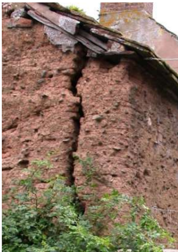
Severe cracking at the corner of this clay dabbin
