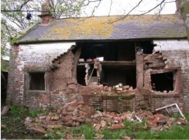
Clay dabbin which was faced with brickwork. The upper floor was inserted at the beginning of the 18 th Century. Uninhabited for some time, the front wall recently collapsed exposing the interior.
