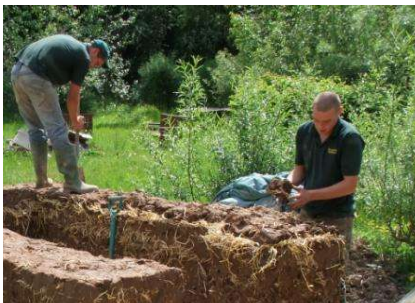
Layers of clay dabbin mixture used to construct the wall
