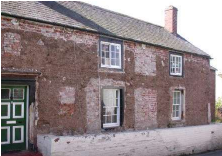
Removal of render will often reveal evidence of earlier alterations to the building. Cross Farm, Burgh by Sands
