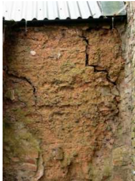
Minor cracking
