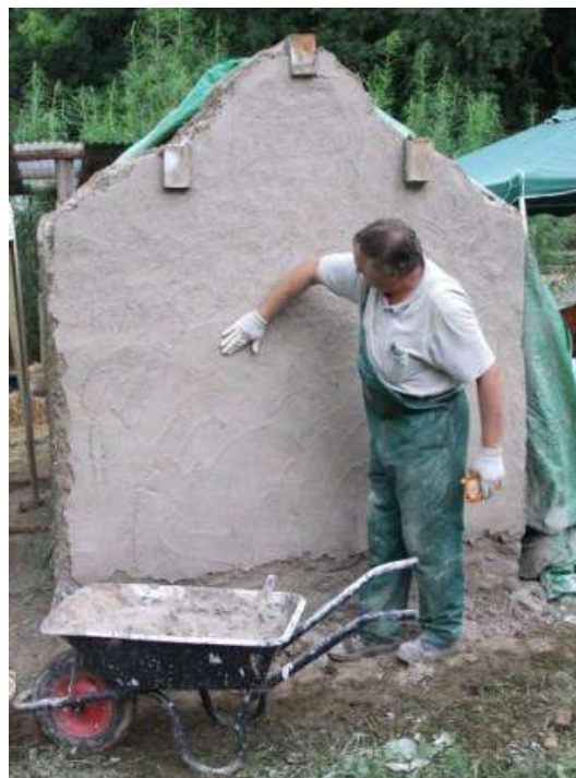
Lime render as finishing coat
