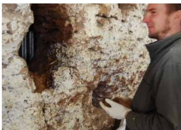
Large hollow in the clay wall
