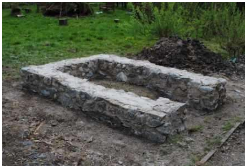
Stone plinth to prevent ground water damage to the base of the wall
