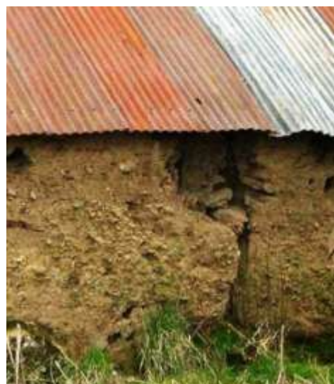
A major crack made worse with a roof with no gutter
