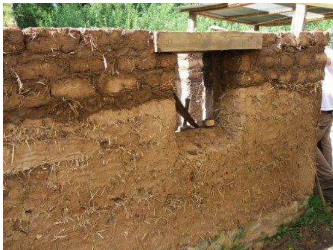
Above and below: Planning the window openings by measuring the height and inserting the timber lintels into the correct location and continuing to construct the structure
