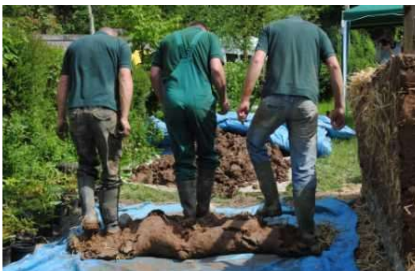
Treading the turned mix, heeling it well in and spreading it out before adding more straw
