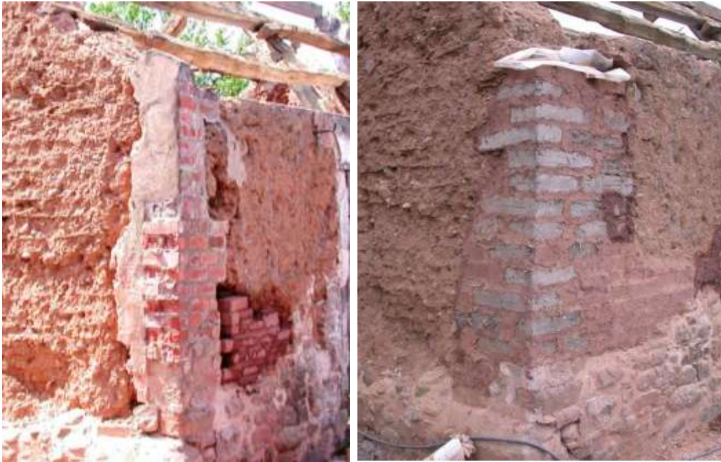
Above: Cracking on the corner of this building was originally repaired in brick with cement mortar. The much harder mortar led to erosion at the junction with the clay, creating cavities and making the wall unstable again. The repair was carried out using clay blocks and a dabbin mix for mortar.
