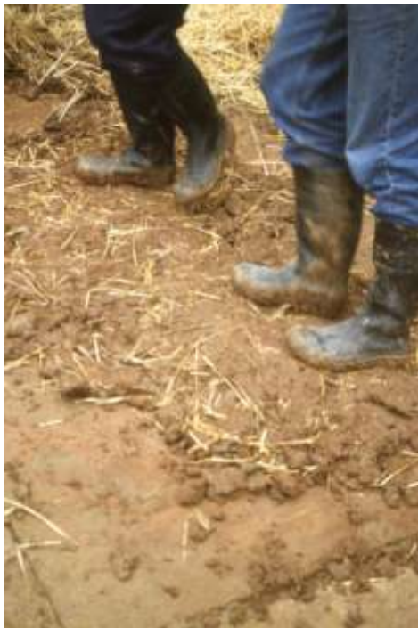
Spreading straw over the wetted clay and using the boot heel to trample it well in
