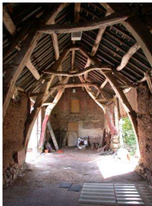
The collars on these cruck frames help to prevent the walls from spreading apart
