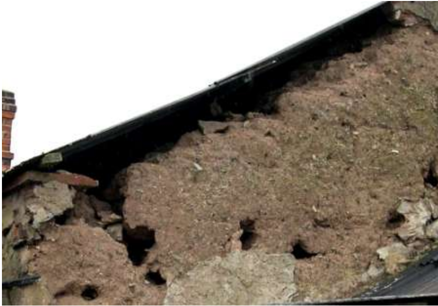
The top of the clay wall is gradually being washed away due to inadequate coverage of the roof.
