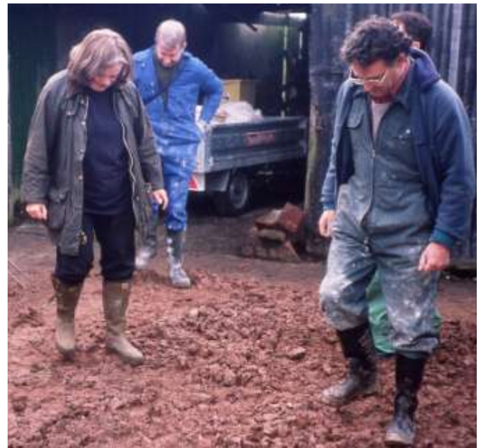
Working on concrete, breaking up the large lumps of clay before adding the straw. Turning it over to ensure it is well wetted through
