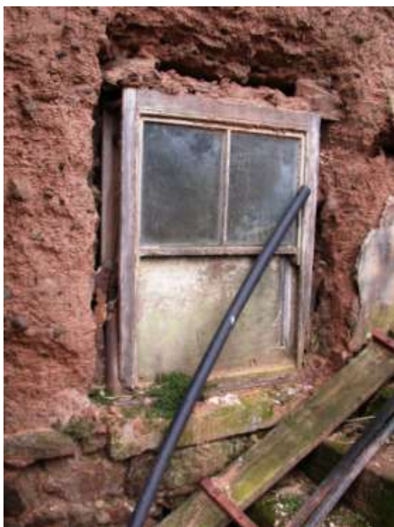
Formerly cement rendered clay wall with sash window set into it. No lintel but a stone sill.
