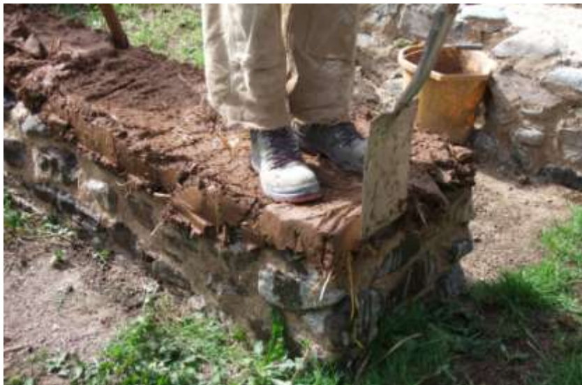
Treading the dabbin and keeping the edge vertical
