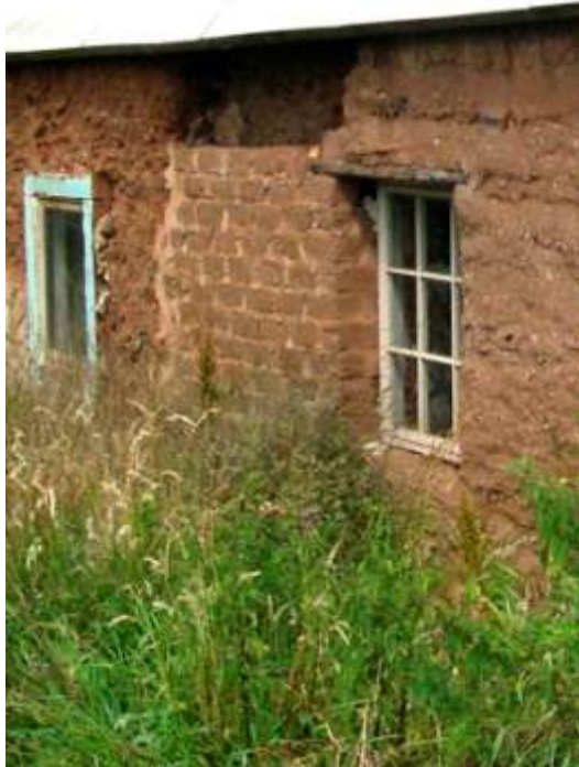
Adding a new clay wall extension to an old clay dabbin, using clay blocks for the junction.
