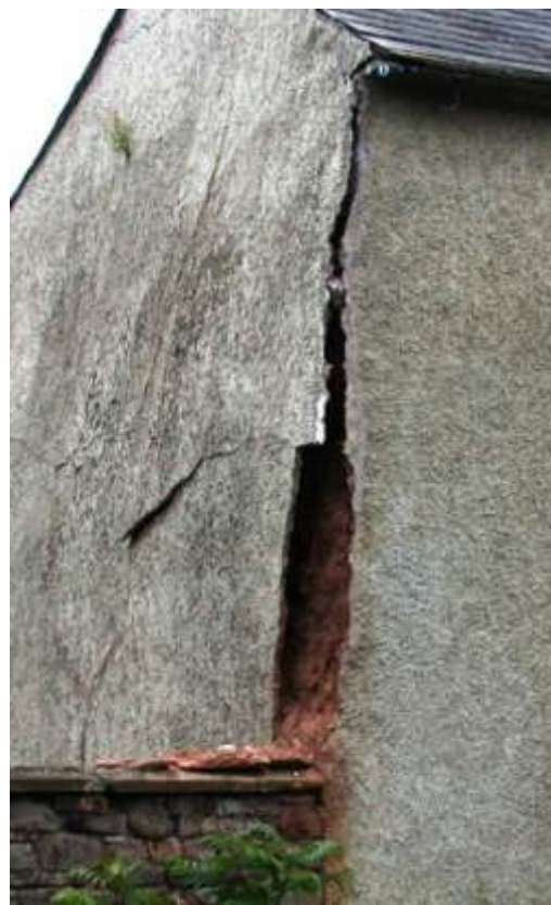
Cement render breaking off the gable of this clay wall
