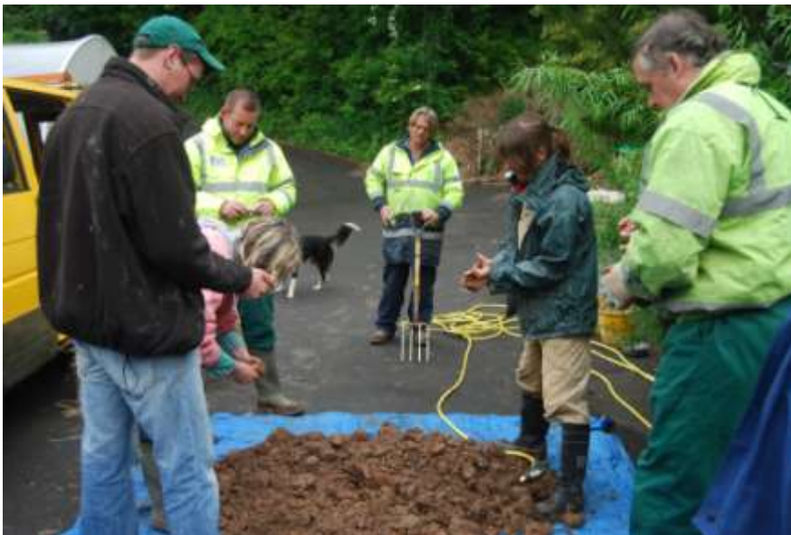
Examining the material to be used in the building, removing any large stones, plant roots and other vegetable matter.
