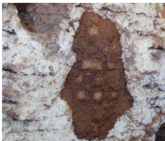
Clay bricks fill the rest of the hollow to create a sound repair
