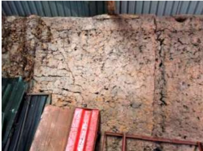
Barn wall showing the junction between old and new clay work. The recess for the post, to which shuttering was fixed, is to the right.
