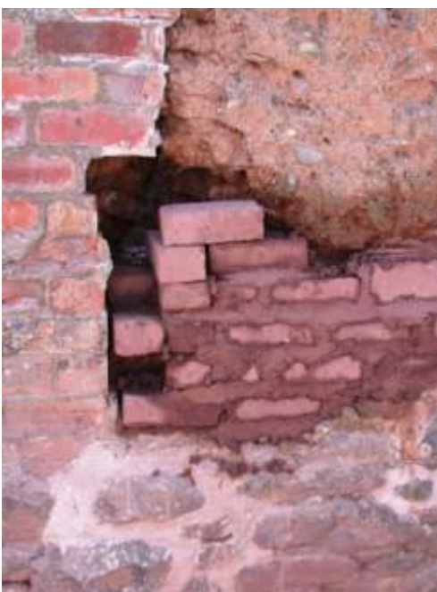
Left: The first stage is to stabilize the adjoining clay wall by underpinning the original dabbin with clay blocks. Later this work can be tied into the repairs on the corner.
