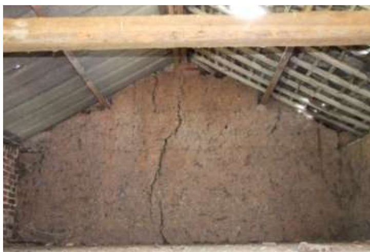
Cracking near the centre of the clay gable wall suggest that the side walls have started to move apart
