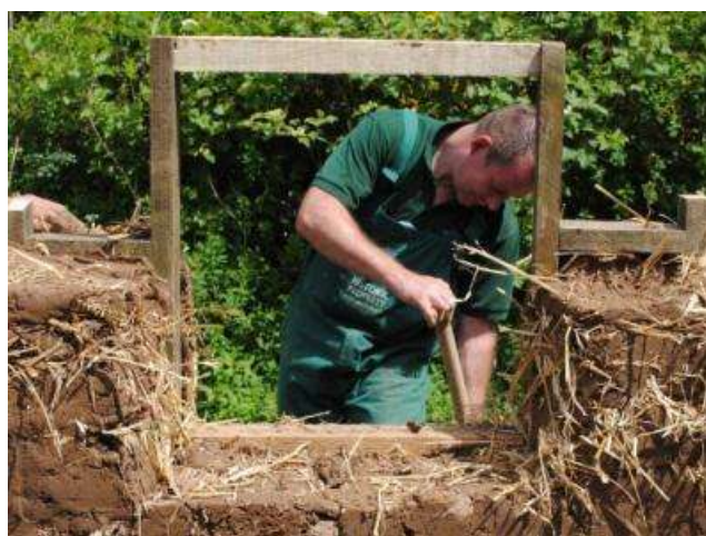
Above and below: Planning the window openings by measuring the height and inserting the timber lintels into the correct location and continuing to construct the structure
