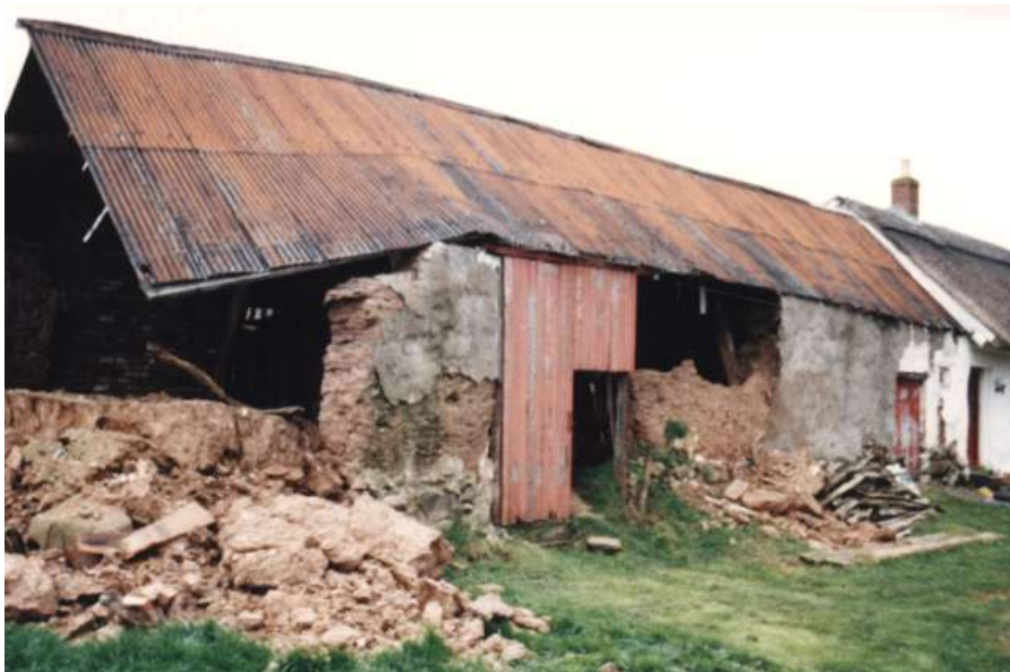
Cement rendered clay wall, trapped moisture was probably responsible for its eventual collapse
