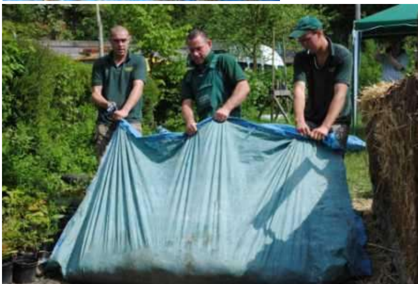
Turning the mix over by rolling it in the tarpaulin
